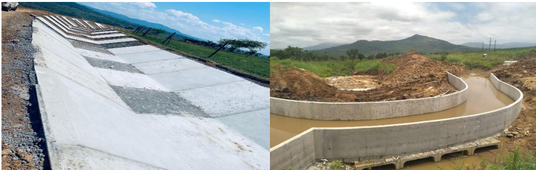
Figure: Ferrera Canal
